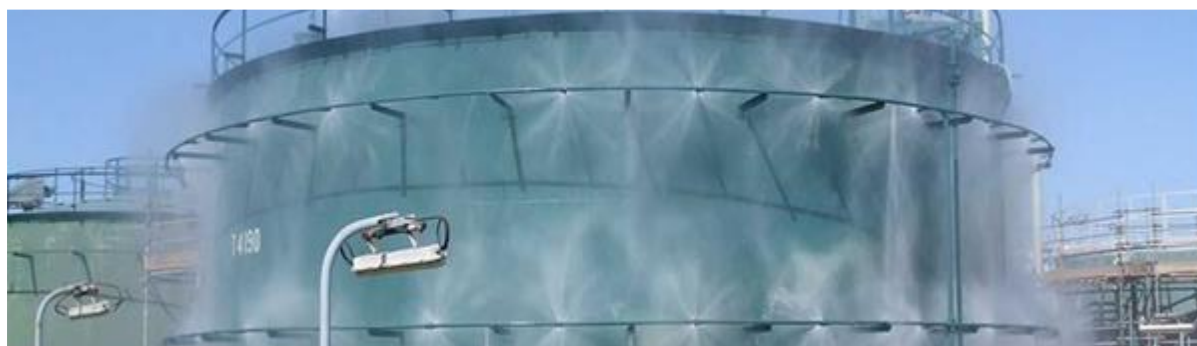
Figure 7. Water Spray System
