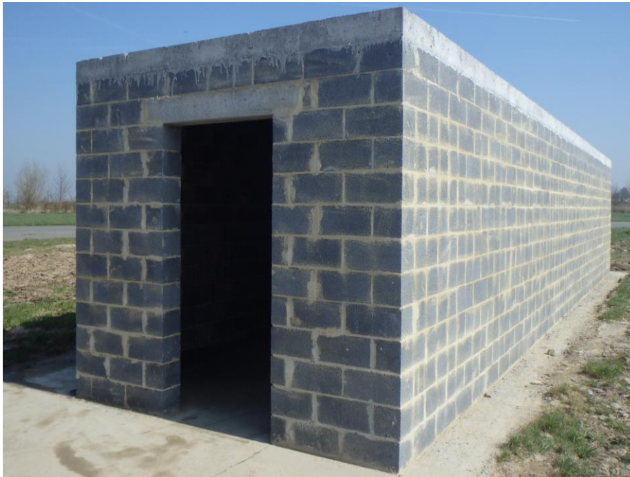
Fig. 5.1 Picture of the skeleton of the construction with concrete bricks.
