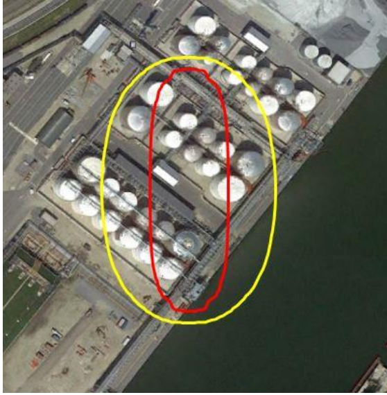
Figure 26. Case study jet fire contours, leakage case
