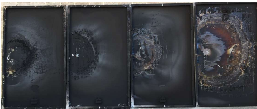
Figure 21 The damaged area of PV panels after the tests (back view). From left to right: tested repeatedly, Test 23, Test 24, and Test 10
