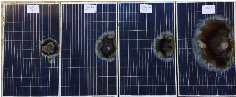
Figure 20 The damaged area of PV panels after the tests (front view). From left to right: tested repeatedly, Test 23, Test 24, and Test 10
