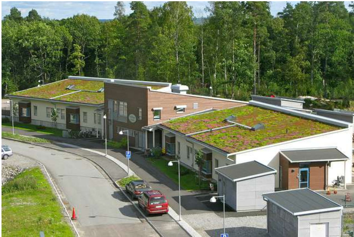
Figure 2.2: A view on the newly built school.
