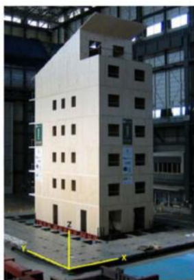
Figure 1.6: Seven-storey CLT building on the 3D shake table [7]
