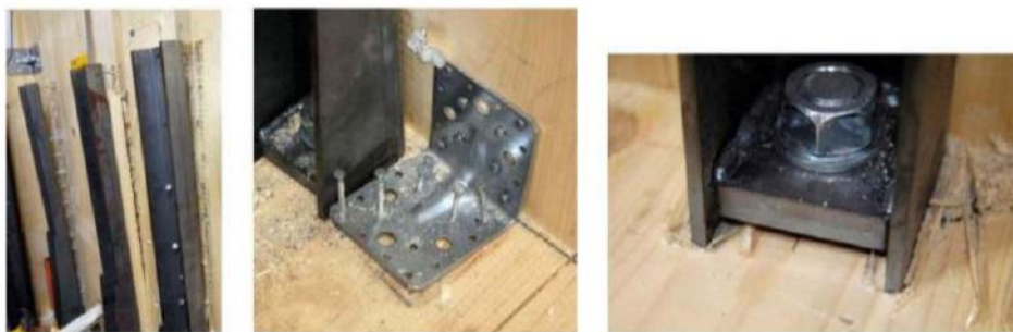
Figure 1.9: Fastener failure of hold-downs (left) pulling-out of nails (mid) wood failure in compression perpendicular to the grain (right) [7]
