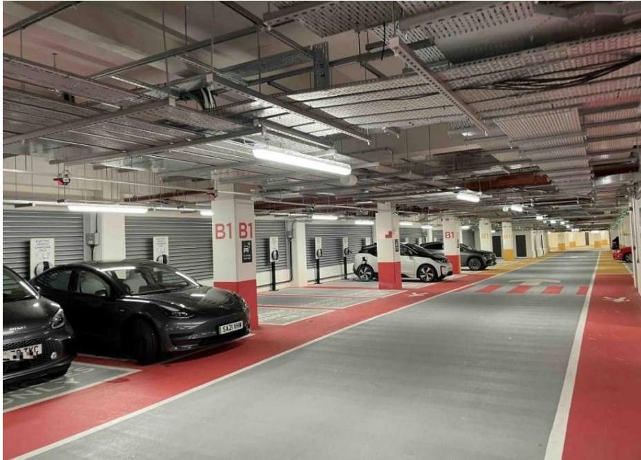
Figure 29: Typical car park with charging facilities
